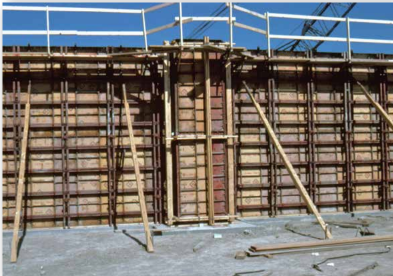
Pilaster Formed with Standard Steel-Ply Components
