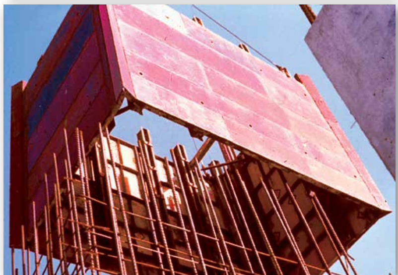
Double Hinged Filler with 90° Inside Corner
