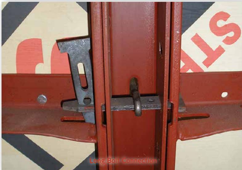
Typical Wedge Bolt Connection
